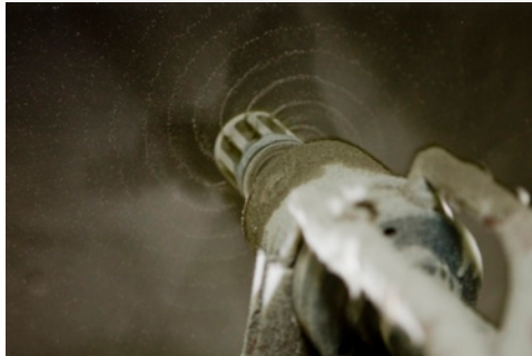
The EcoCast spray applicator spins at 5000 RPM when applying GeoSpray to the line's surface.
