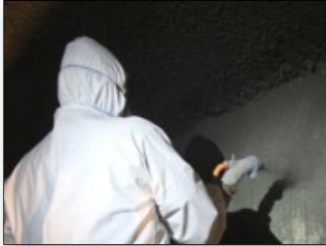
High pressure hoses dispense GeoSpray
