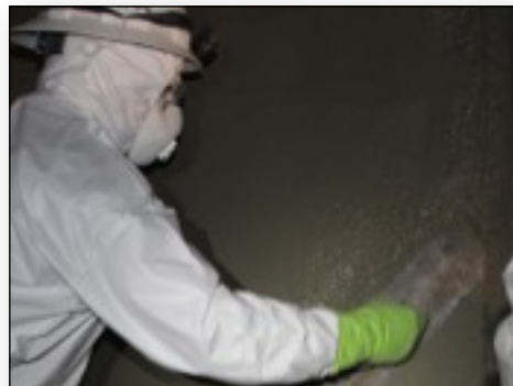
Trowels are used to smooth the finish on flat surfaces
