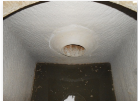
Same manhole renewed with EcoCast Advanced Geopolymer Lining System.
